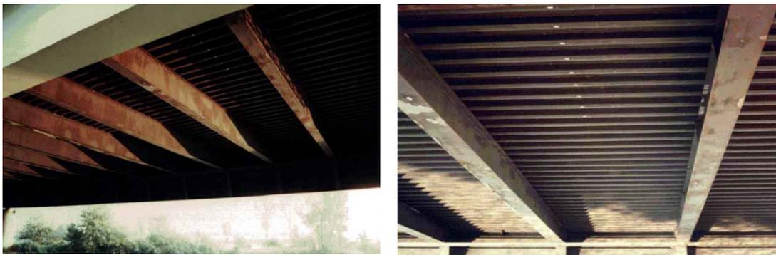
Figure 58: Details of transverse cross beams supporting the longitudinal stiffeners and instrumentation
