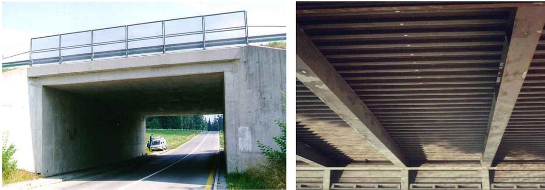
Figure 48: FAD installation on a short slab bridge (left) and instrumented section of the orthotropic deck bridge in Autreville (right)
