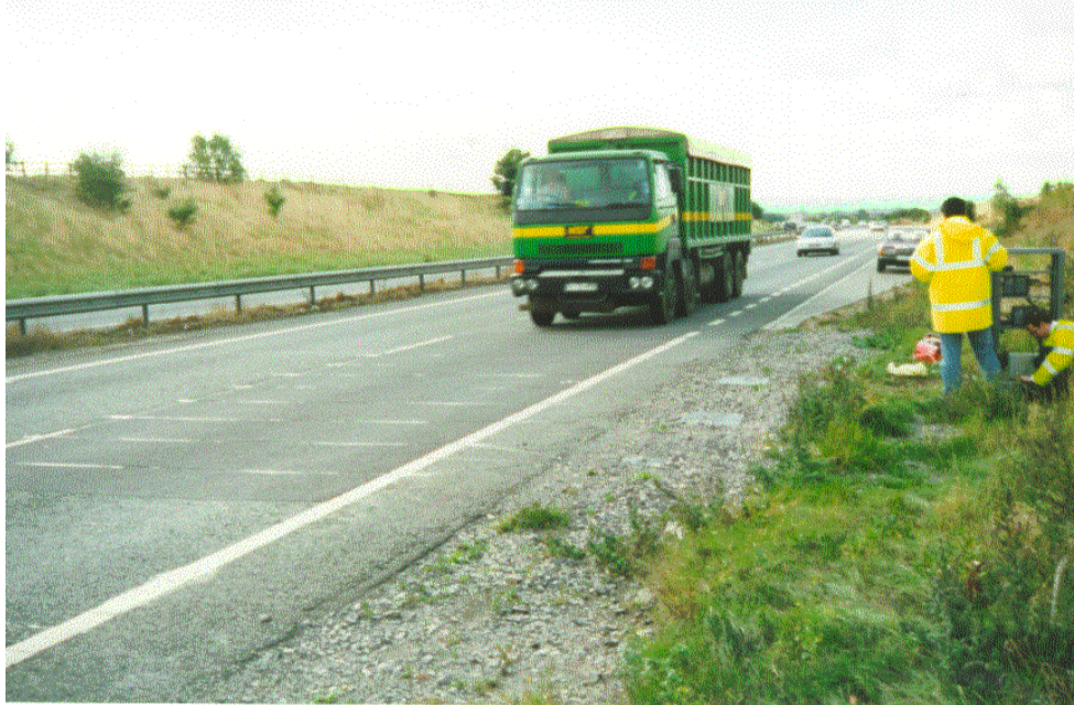
Fig. 31 Completed MS-WIM installation on the A34.
