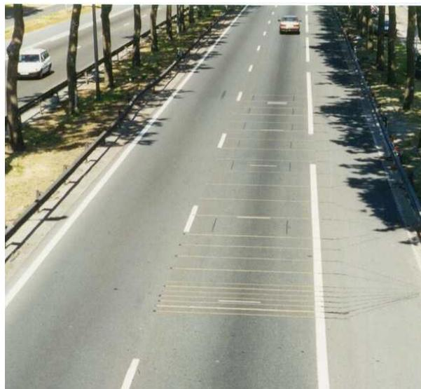
Figure 7: Picture of Trappes MS-WIM array, RN10, France
