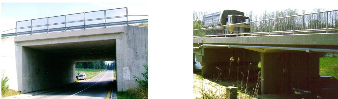
Figure 20: Two types of slab bridge instrumented for bridge WIM
