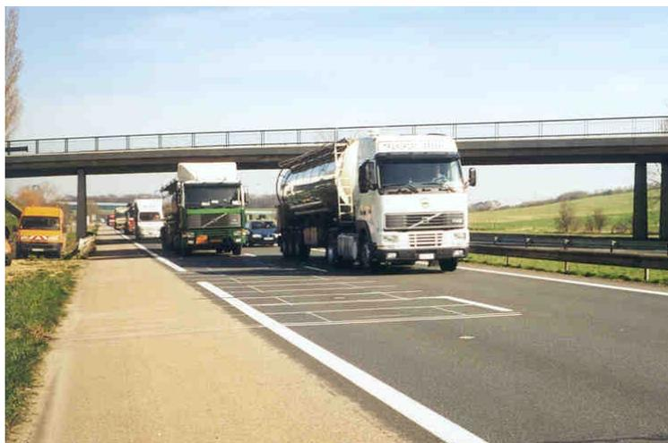
Figure 8: Picture of Metz MS-WIM array, A31, France
